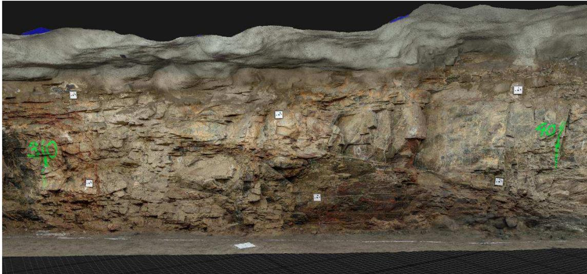
Figure 2. Textured mesh of a 360-degree camera-based photogrammetric model improved by adding extra DSLR images of the tunnel wall.
